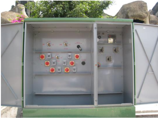
Three phase Pad-mounted Transformer
